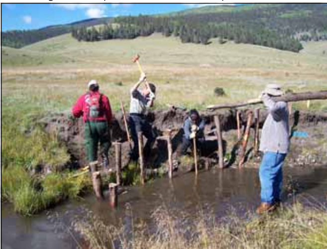
The Santa Clara fire crew install a vane with a J-hook to help protect an eroding bank and provide RGCT habitat, September 2006.
