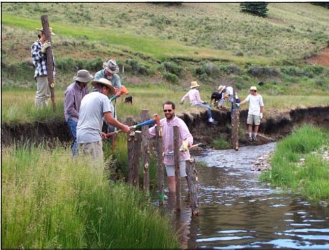
AWF Volunteers build post vanes along eroding banks of Comanche Creek, July 2005.
